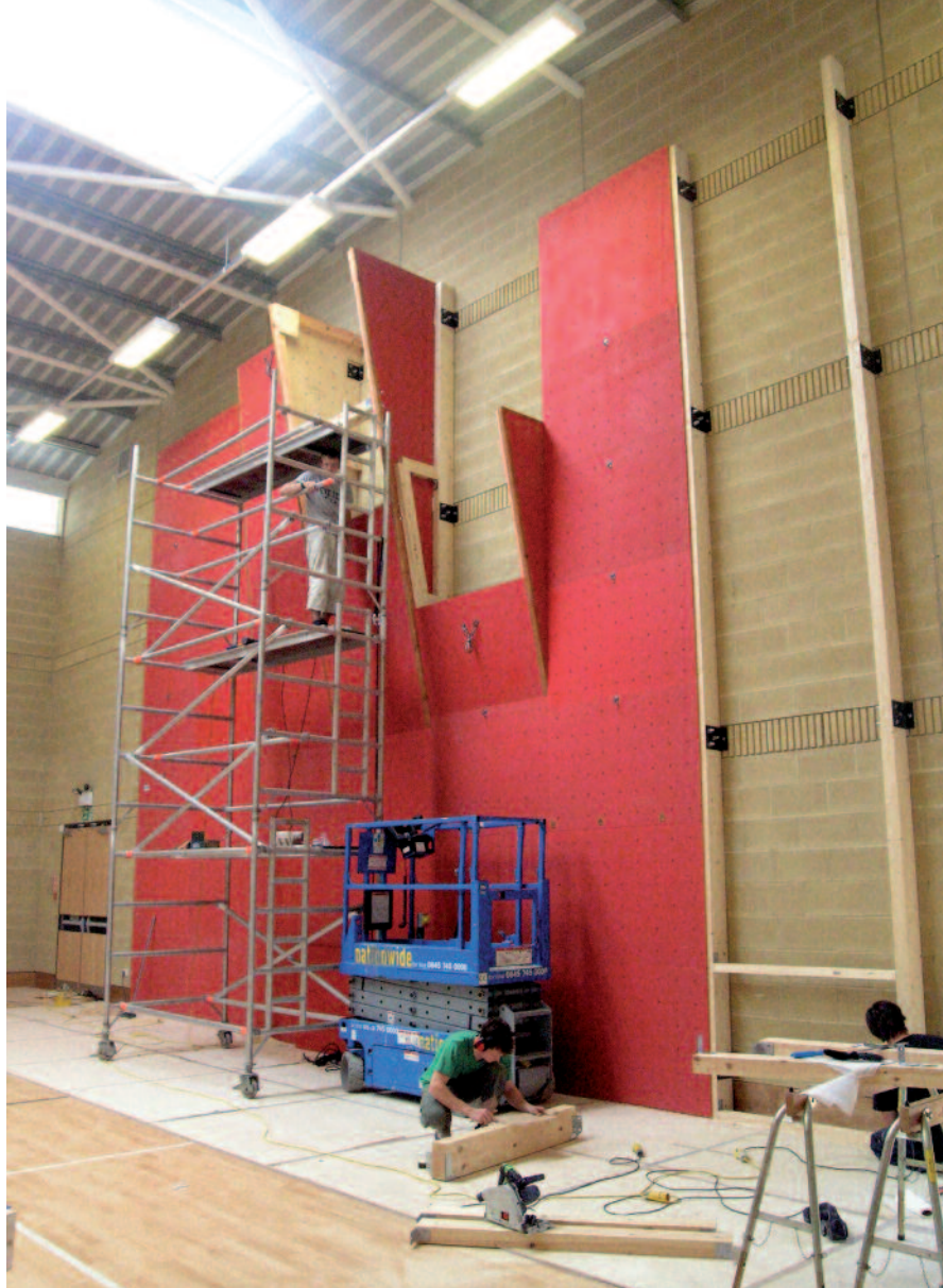
Photos courtesy of Entre-Prise UK.
